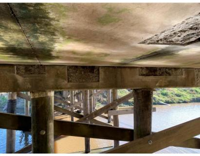
LIGHT-WEIGHT CONCRETE AND POPCORN + LACK OF SEALING CAUSES:
