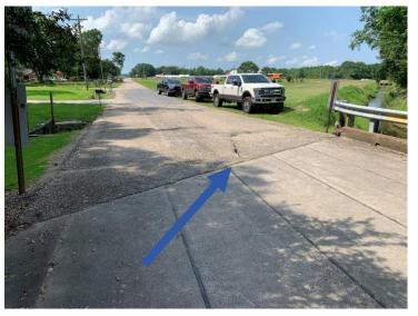
Approach Slab extends directly from Clear Width.
